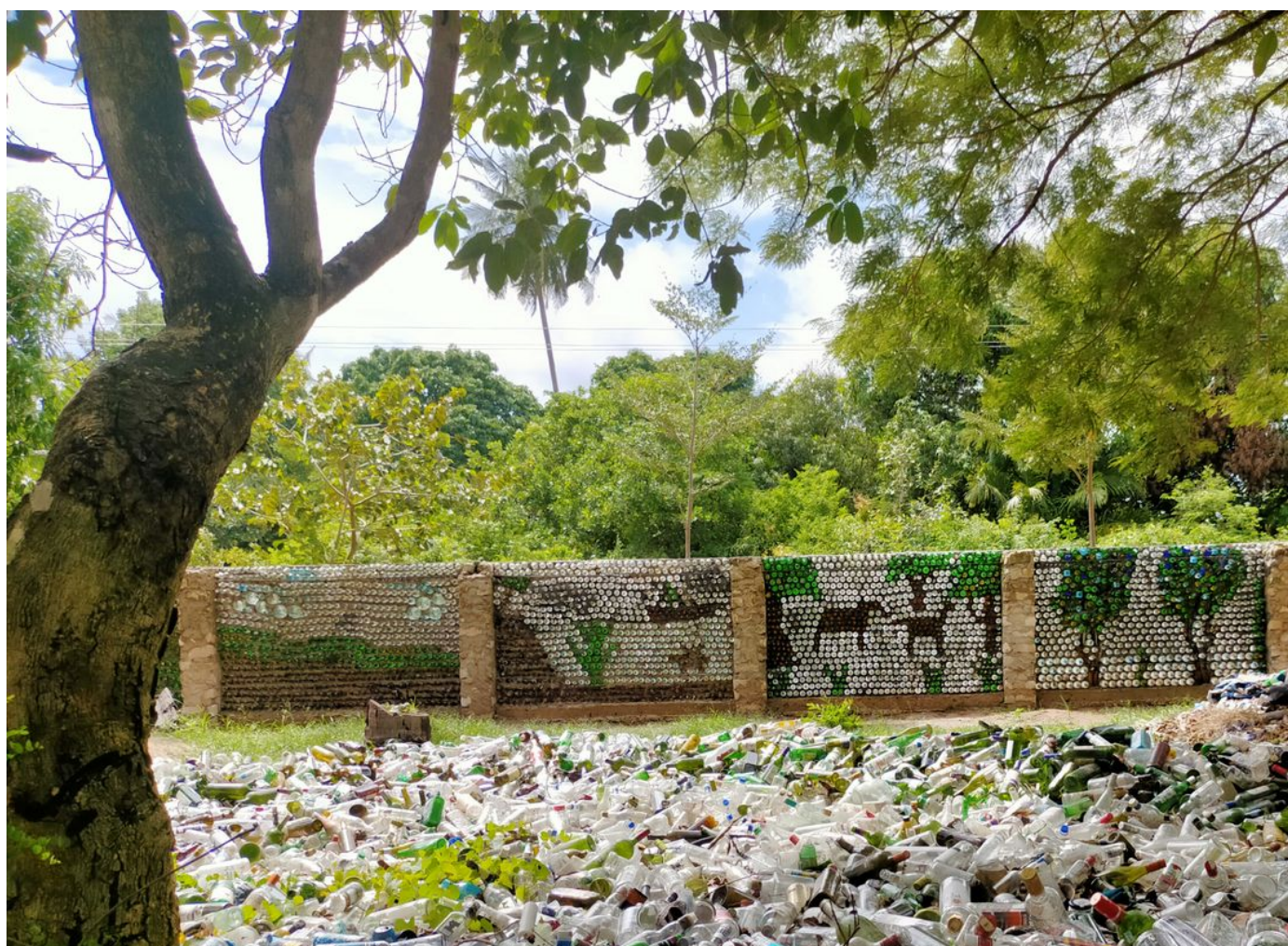
Wall made from old glass bottles in Kenya
